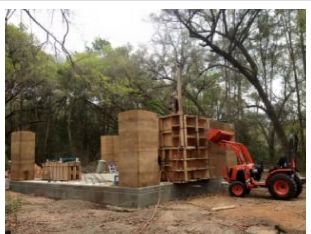
filling the formwork – Johns Island Rammed Earth home
