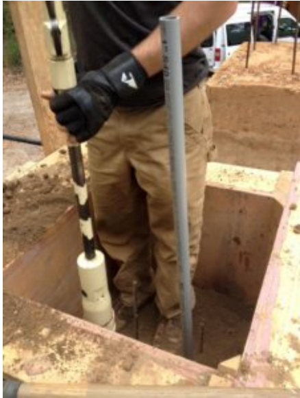
tamping (ramming) the earth mix
